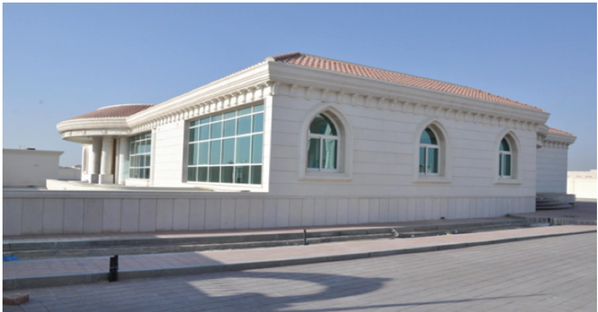
B+G Majlis Block for Mr. Faraj Ali Bin Hamoodah-Exterior view
